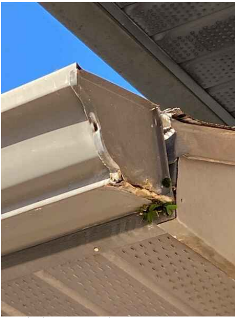
Corroded gutter end cap
