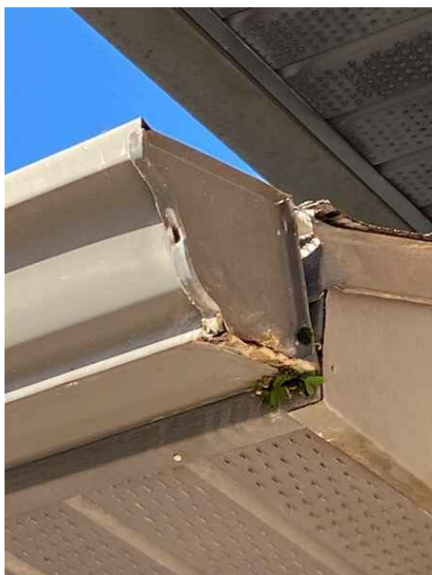
Crooked gutter end cap
