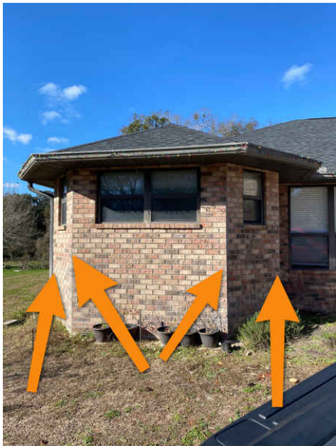
East side of house Masonary should be evaluated for repointing
